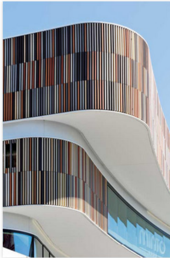
Located in Mönchengladbach, Germany, Minto is a vibrant shopping mall. Designed by Kadawittfeldarchitektur, the project consists of vertically installed baguettes in a variety of natural terra cotta colors.
